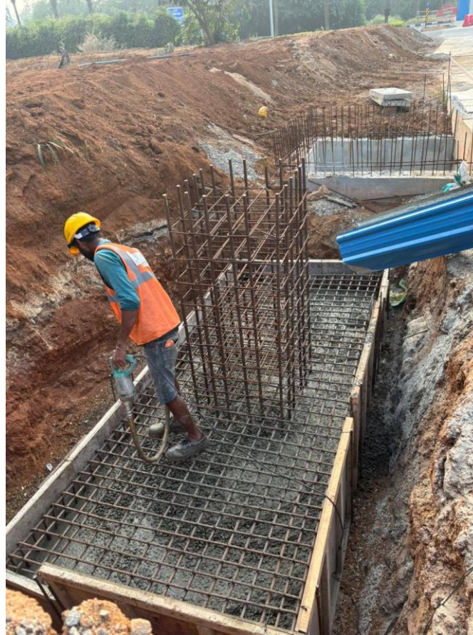
Construction of Footings for Gantry at Hyderabad International Airport Main Access Road (GMR Work)
