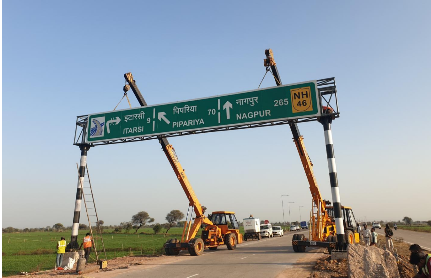
Fabrication and Installation of Over Head Gantry on Obedullagnj-Itarsi NH-46 Section
