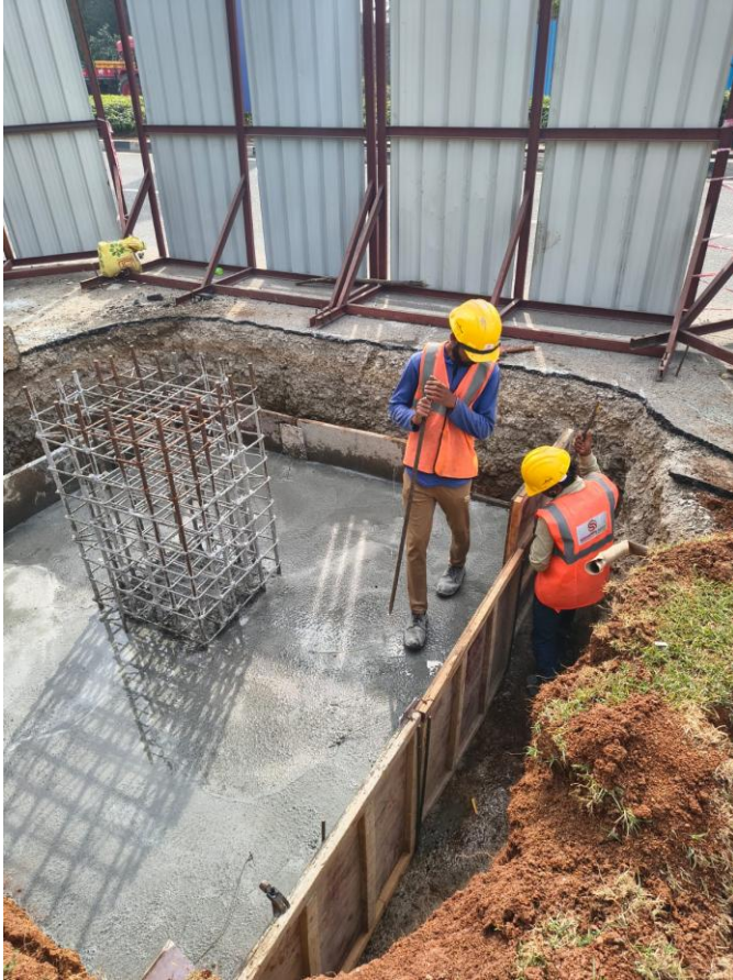
Construction of Footings for Gantry at Hyderabad International Airport Main Access Road (GMR Work)
