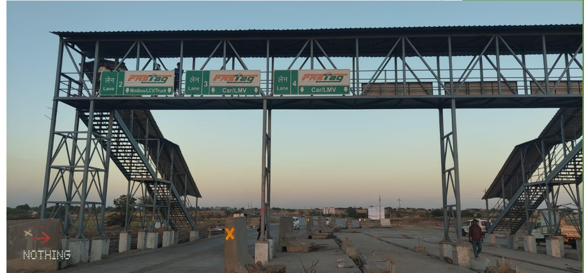
Fabrication and Erection of Foot Overbridge at Toll Plaza and Installation of Toll Plaza Sign boards on FOB at Mohol-Wakhiri NH Road
